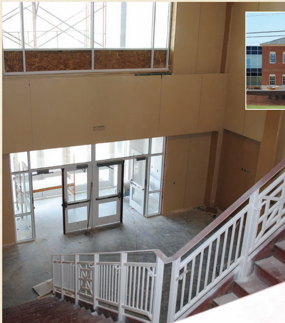
View from inside front entry – exit toward Trimble Road.
